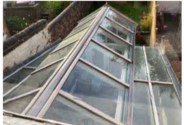
Existing View from 1 st Floor Bedroom Window
