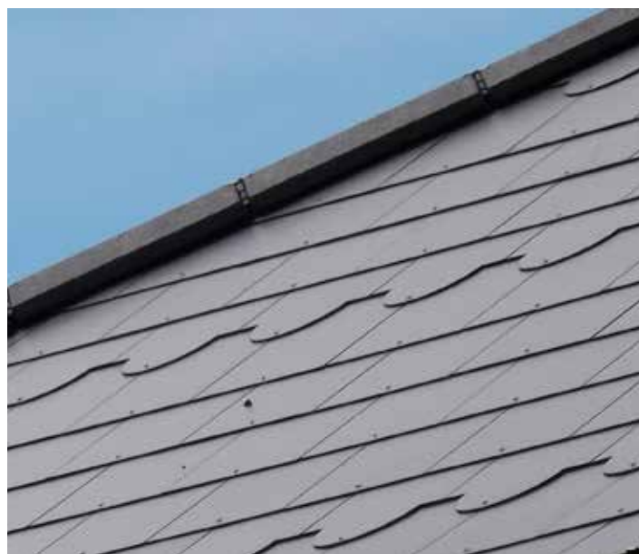
Continuously ventilated monopitch ridge
