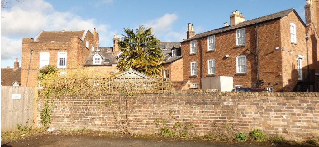
The design provides a low silhouette in the rear views of the site
