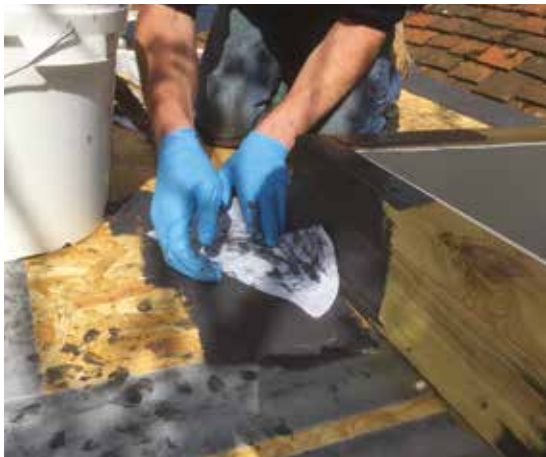
Detailing to roof light reinforced with fabric
