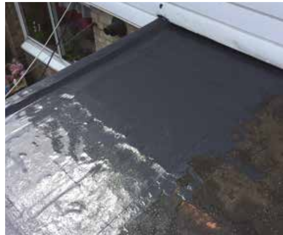
Apply FIX-R Fabric to reinforce
