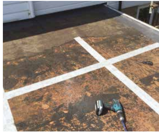
Prepare the surface: Use jointing tape to cover joins in the surface
