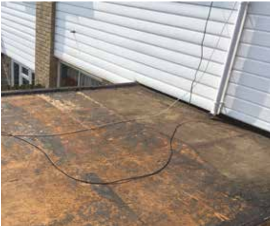
Surface before application
