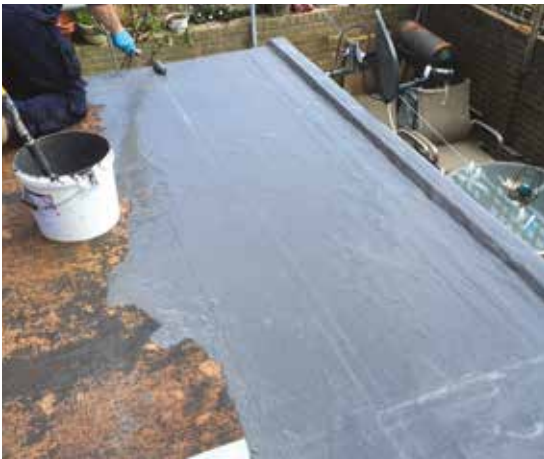
Apply FIX-R Liquid Waterproofing
