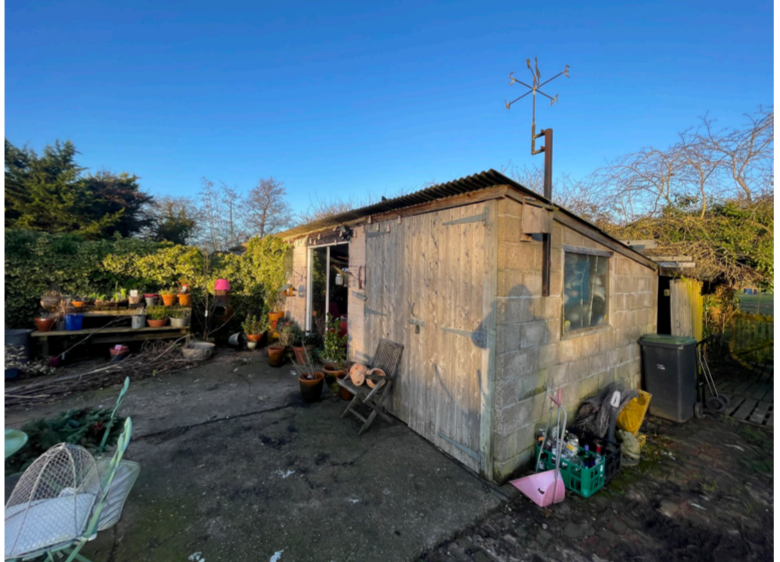
VIEW 02 - East and South Elevation of existing Outbuilding to be replaced
