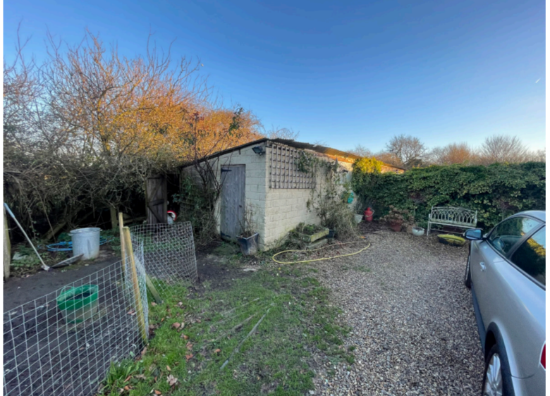
VIEW 02 - West and South Elevation of existing Outbuilding to be replaced
