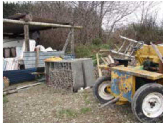
Photo 5: temporary roofed area in front of cutting
