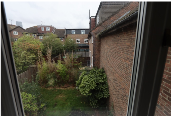
View of existing garage wall from FF.
