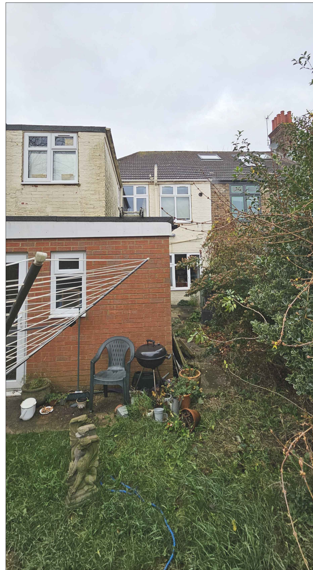
Photo 1 - Rear of no.1 @ 1:50
