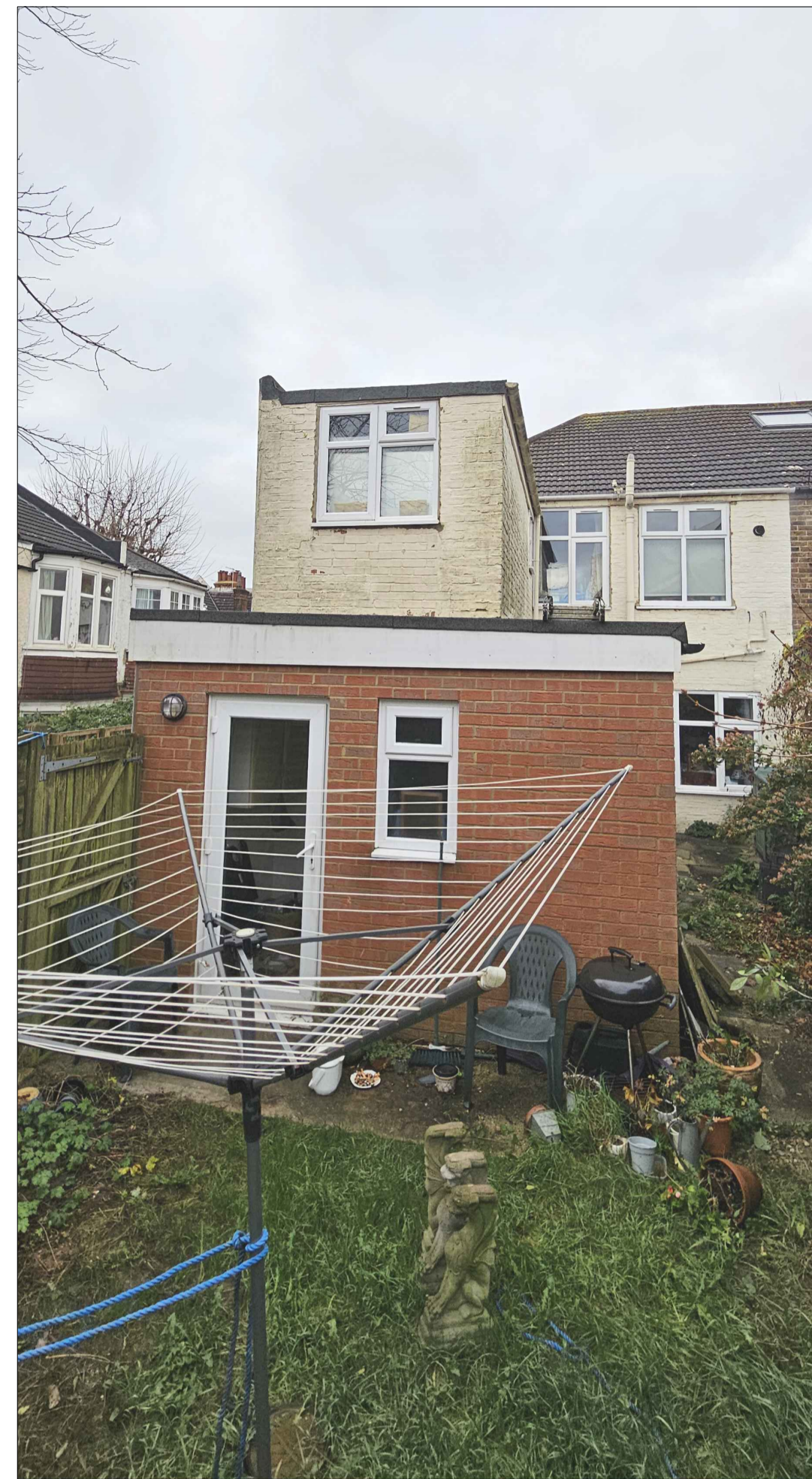
Photo 2 - Rear of no.1 (red brick extension to be demolished)
