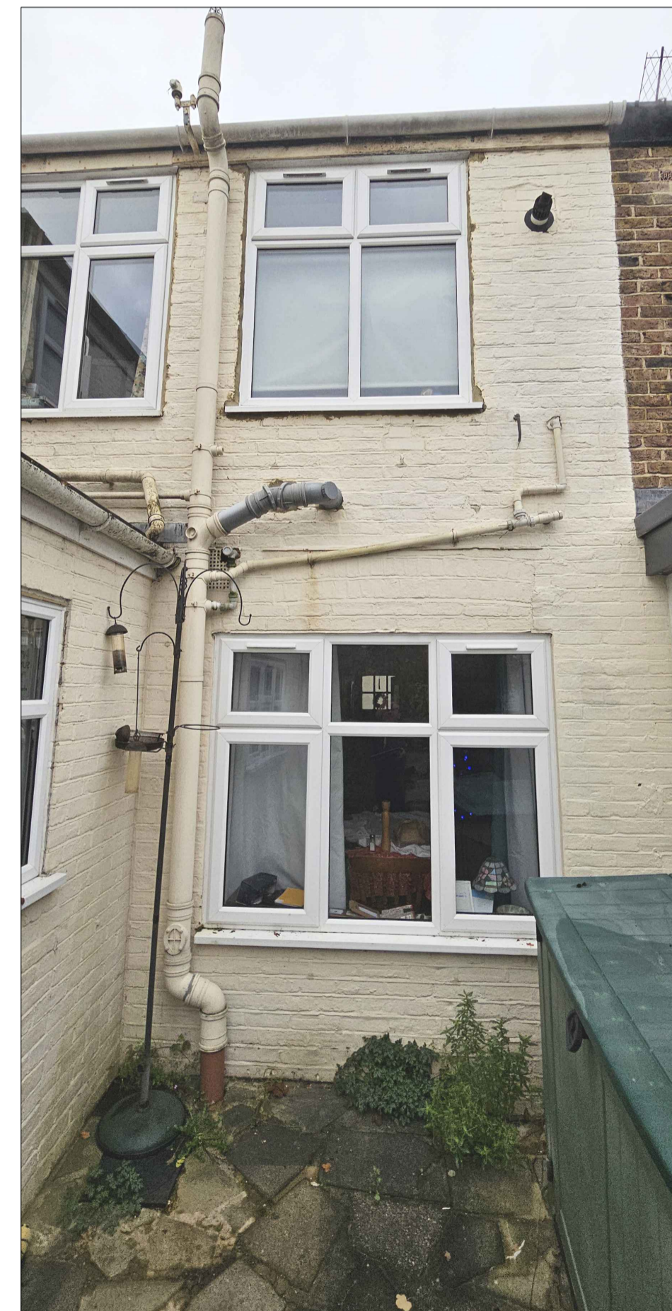
Photo 6 - Rear of no.1 side return
