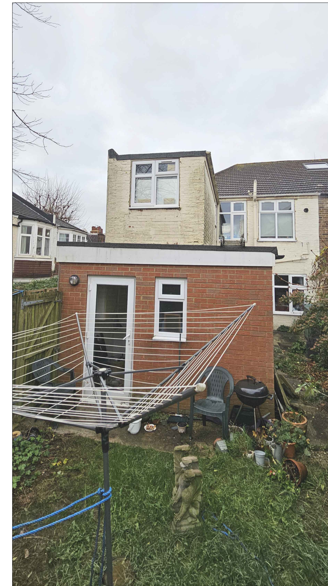
Photo 4 - Rear of no.1
