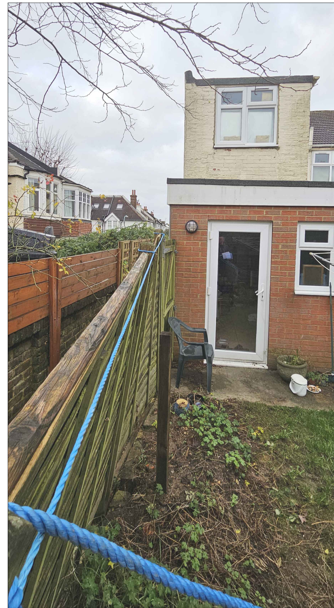
Photo 3 - Rear of no.1 - alleyway access to left of photo
