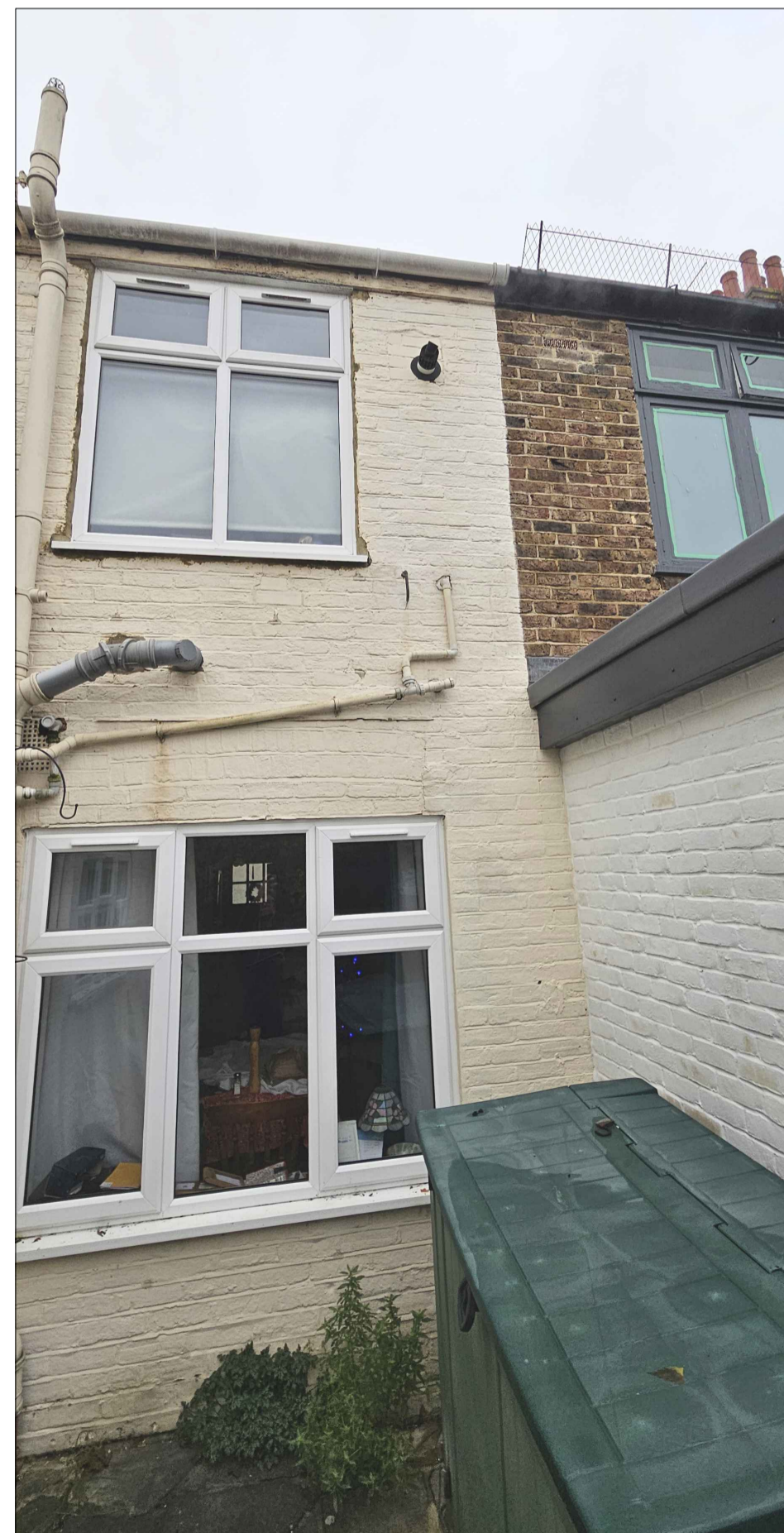
Photo 5 - Rear of no.1 side return
