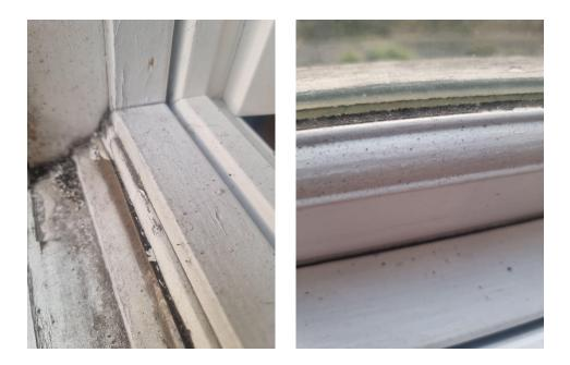
Additional plates have been added to the casement to reduce draughts. The second photo shows the sharp moldings to the windows and the seals that have deteriorated internally.
