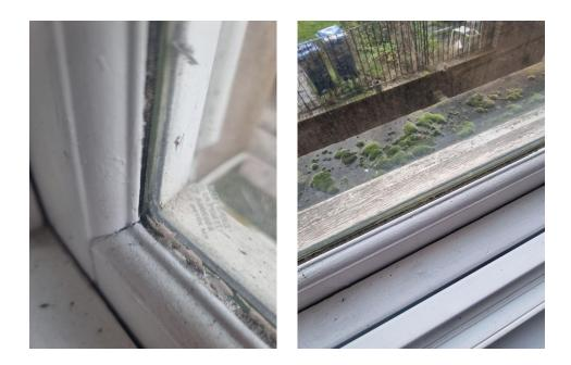
The seals around the glass internally and externally have deteriorated and therefore the glass is no longer sitting properly within the sash. This is allowing wind to channel through the windows.
