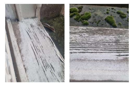
The sills to all windows are water damaged and starting to show signs of rot. The mastic has also come away from the windows which is allowing water to enter the casement.
