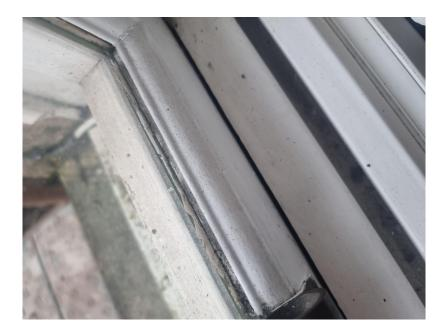
Seals around the glass have come away, allowing wind to enter the property. The glass is not original and the curved bevel on the moldings around the windows show that they are not original and therefore not historically relevant.
