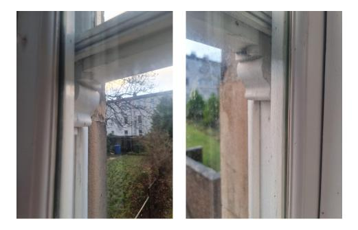
The molding on the horn shows that these windows are not original. This is known as the curvature on top grove nearest the glass is a follow-on of the bevel of the sash. This is something that is only seen on modern windows.
