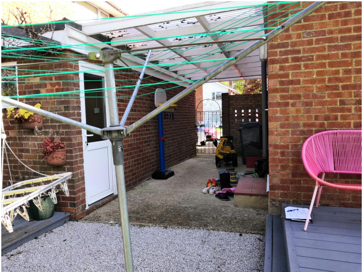
Photograph showing The lean-on area covered the side of the property from rear elevation between the house and the garage.
