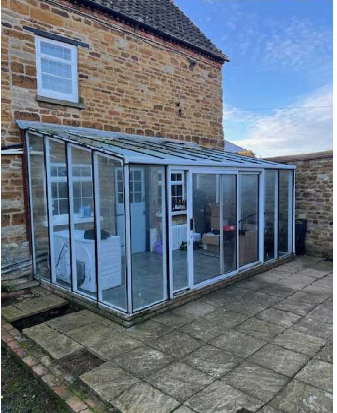
The existing rear conservatory
