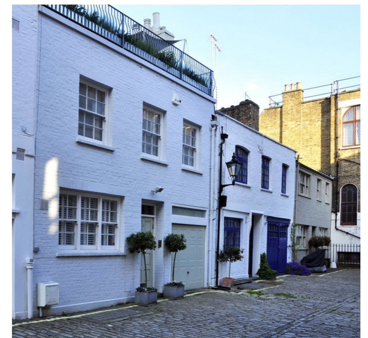
Figure 5.3 Clarkes Mews (The Site is the middle property)
