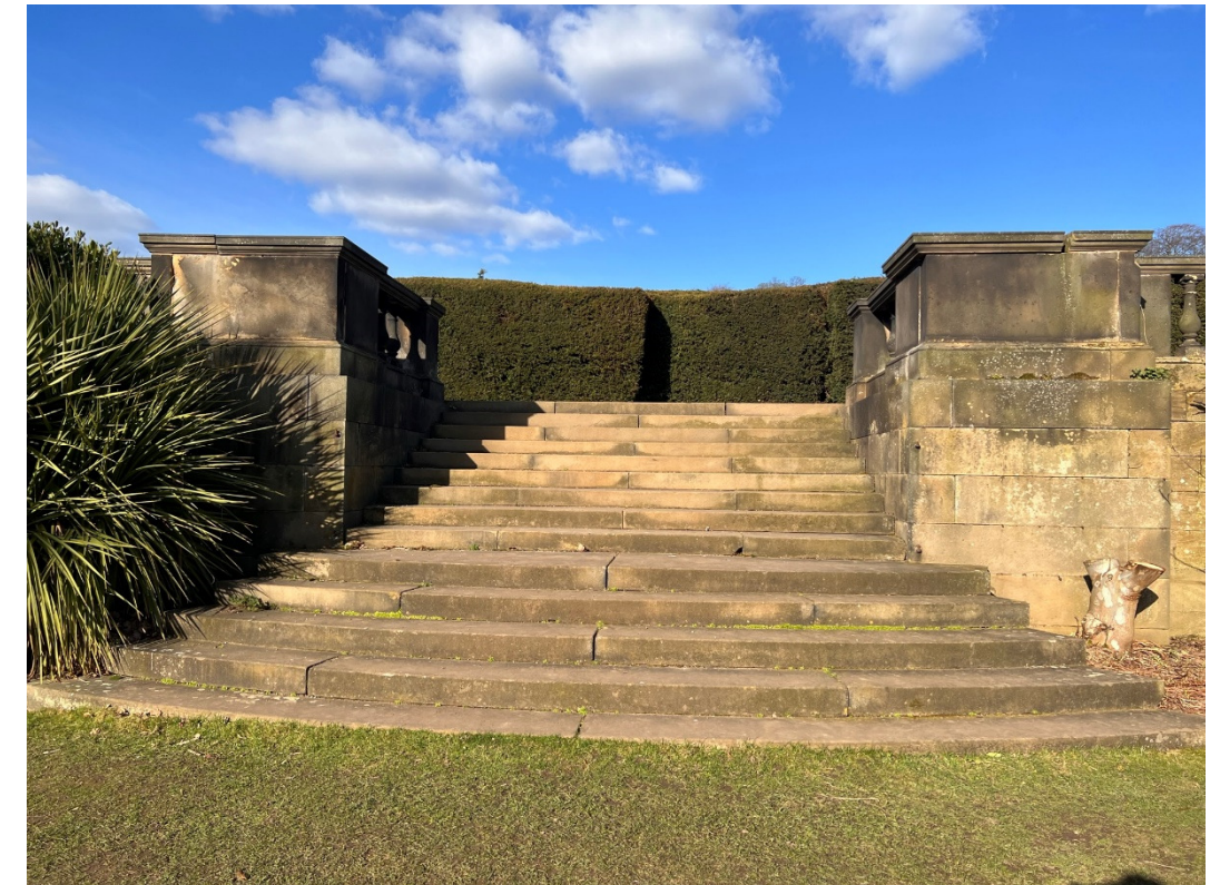
Figure 11 – Typical staircase to Terrace
