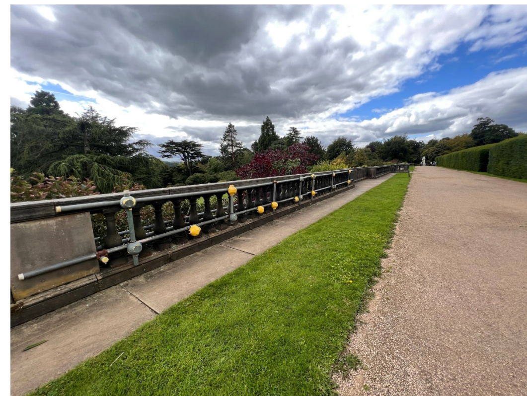
Figure 1 – View of Terrace from East showing temporary scaffolding supports.
