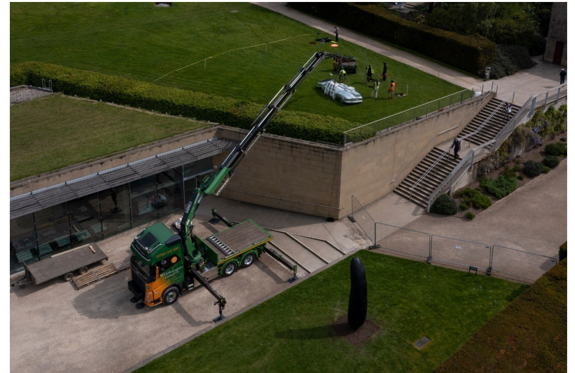
Figure 13 – Image showing typical crane lifting activities at YSP
