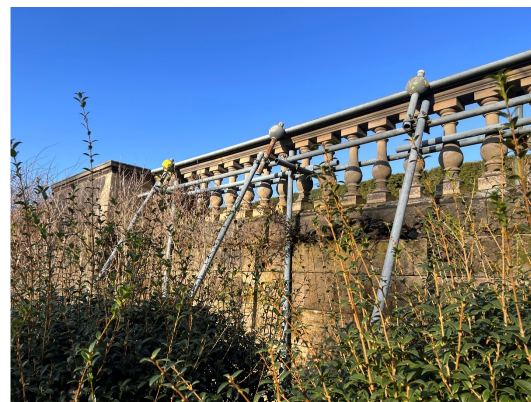
Figure 1 – View of Terrace from East showing temporary scaffolding supports.
