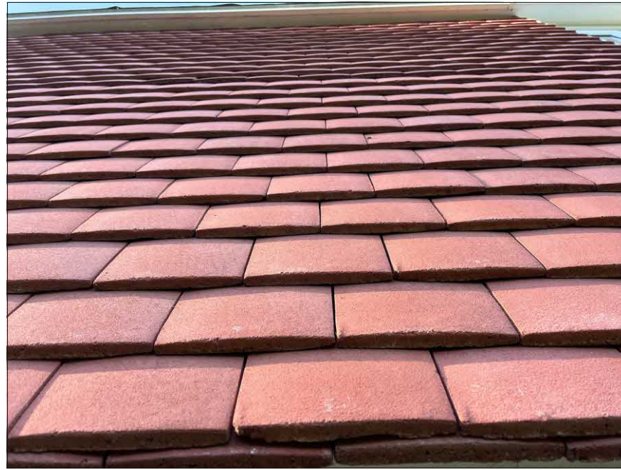
Photograph 2: Showing the close inspection of the well-sealed tile hanging.
