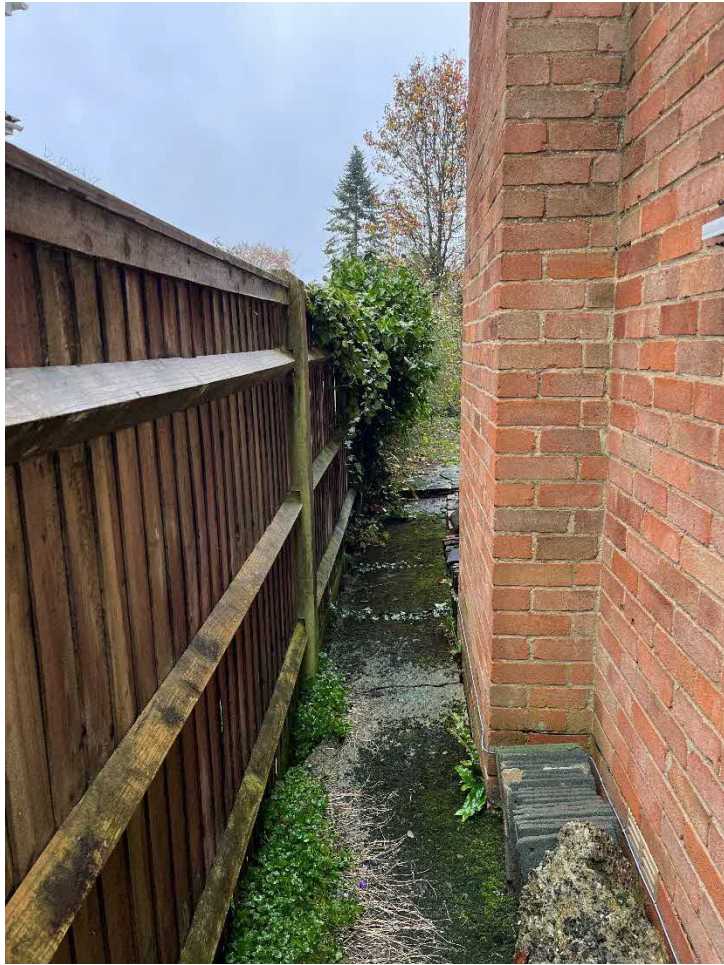
West Elevation looking North
