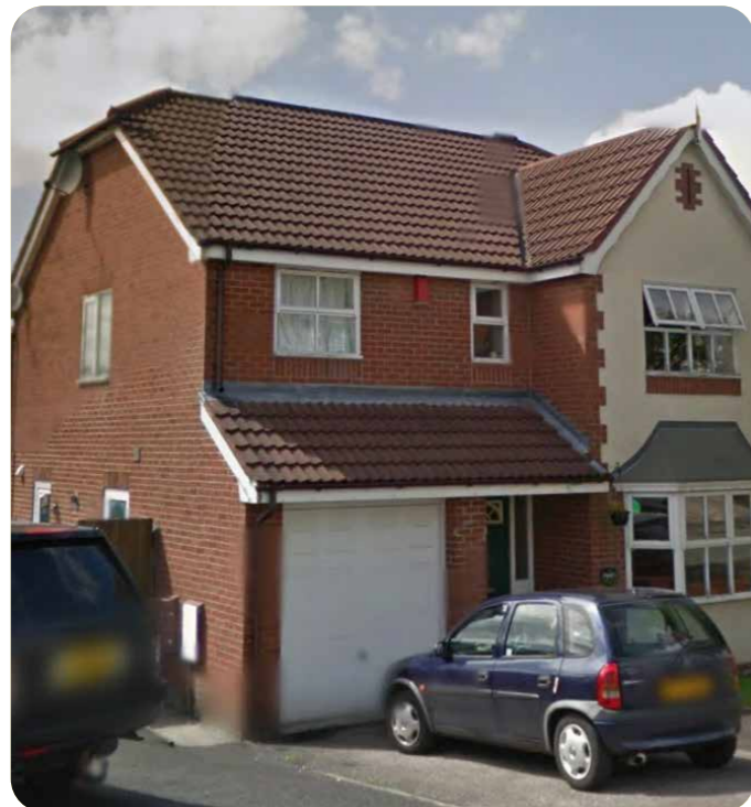
Brick Heads and Cills George Street
