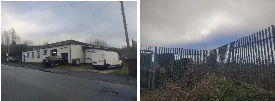
Figure 3: The site as seen from Linney Lane, looking south-east (left) and the south-western site corner with a locked access gate into the Shaw Distribution Centre and the off-site River Beal located on the opposite side of the boundary fence (right).
