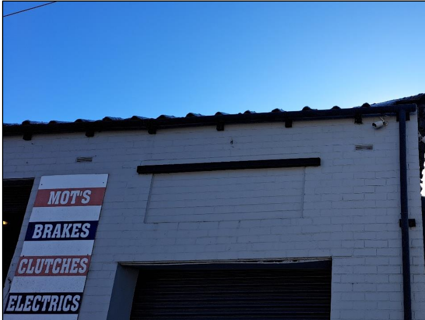
Photograph 2 showing the roof edge
