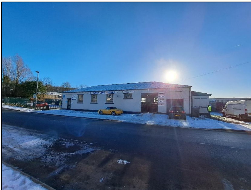
Photograph 1 showing the northern elevation of the building
