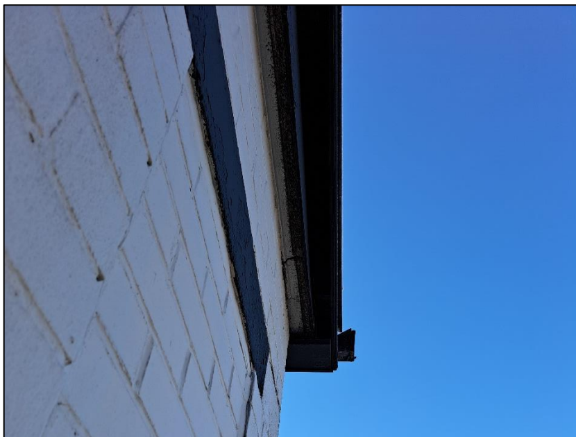
Photograph 3 showing the soffit and fascia on the lean-to
