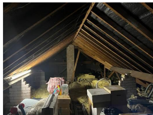
Figs. 8 & 9 Roof voids lined with bitumen felt
