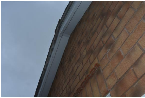
Figs. 5 & 6 Eaves fully sealed/soffits tightly fitting
