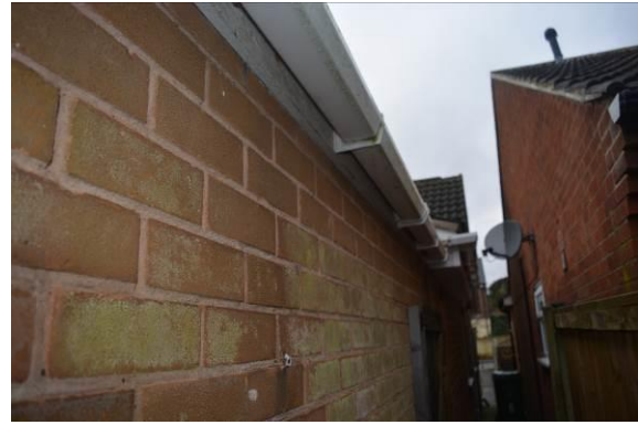
Figs. 5 & 6 Eaves fully sealed/soffits tightly fitting
