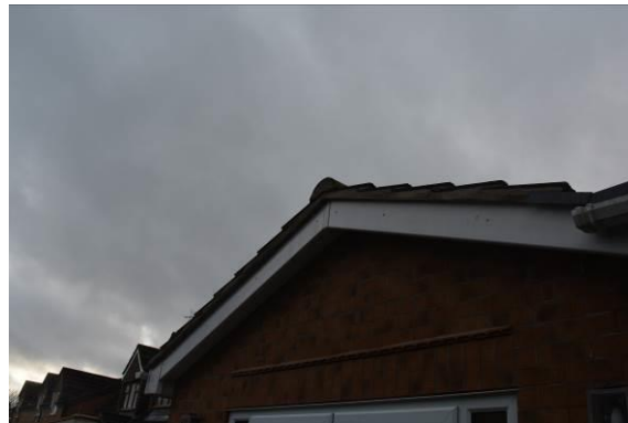
Fig. 7 Gable ends sealed with mortar
