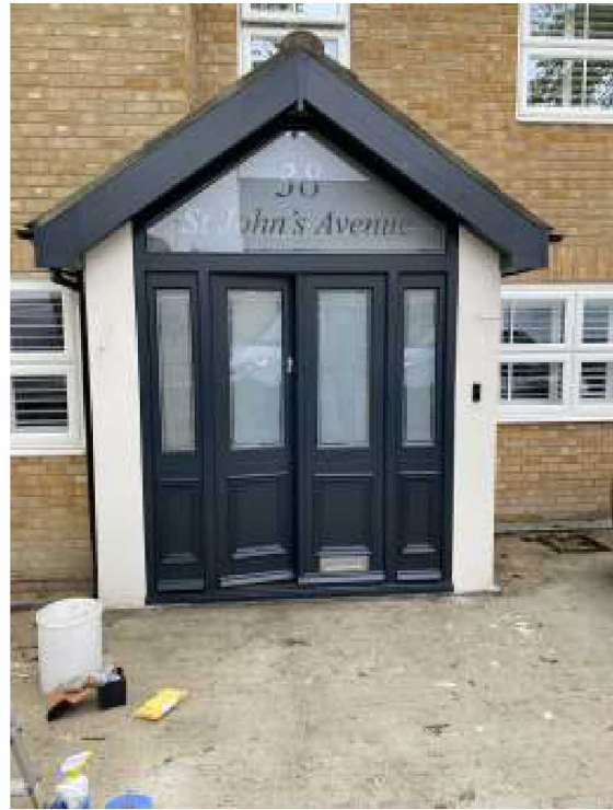
Front Porch view
