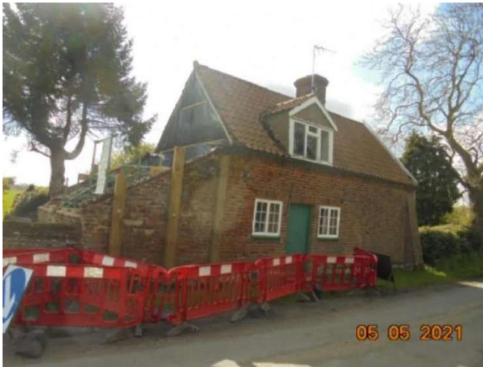
Image above: Clay Lane Cottage on 5 May 2021 prior to demolition
