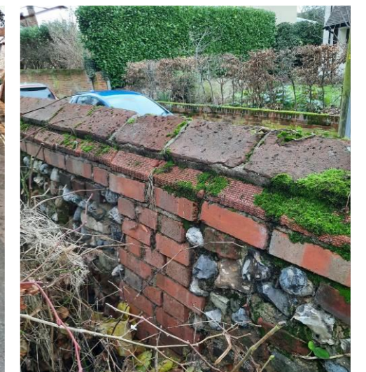
REAR FACE WITH MODERN BRICKS
