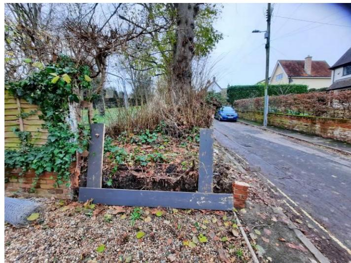
RETURN AT SOUTH END
