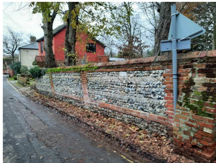
VIEW ALONG WALL LOOKING SOUTH
