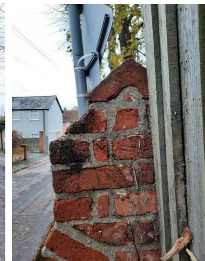
PART VIEW OF COPING
