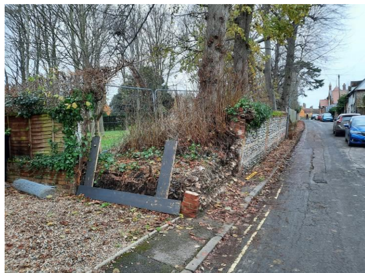
VIEW AT SOUTH END WITH TREE BEHIND
