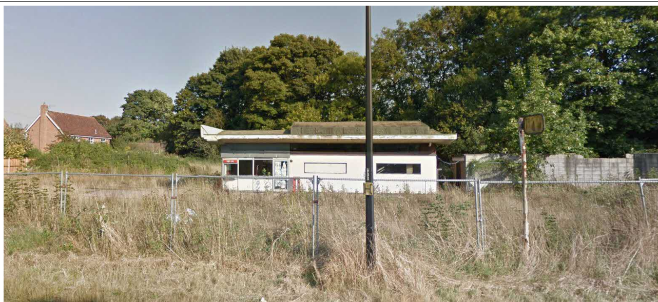
Figure One: The Site Viewed from the Road - September 2016
