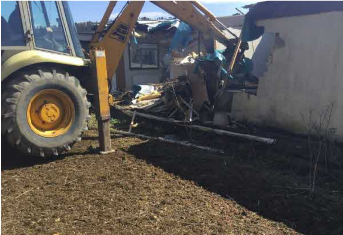
Photo 1 –Demolition of former dwelling on 26th April 2019
