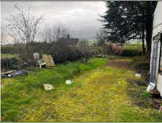
P7: A view of the driveway and northern wall of the cottage facing south-east
