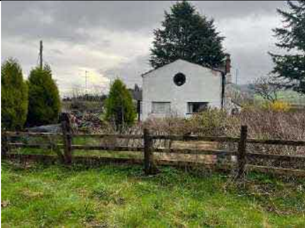
P3: View of limekiln cottage facing east
