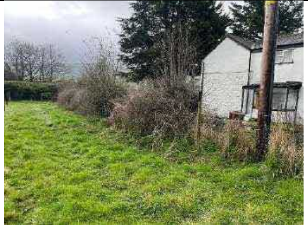
P4: Second view of the cottage facing south-east
