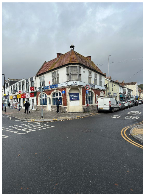
Figure 1. Images of the existing building
