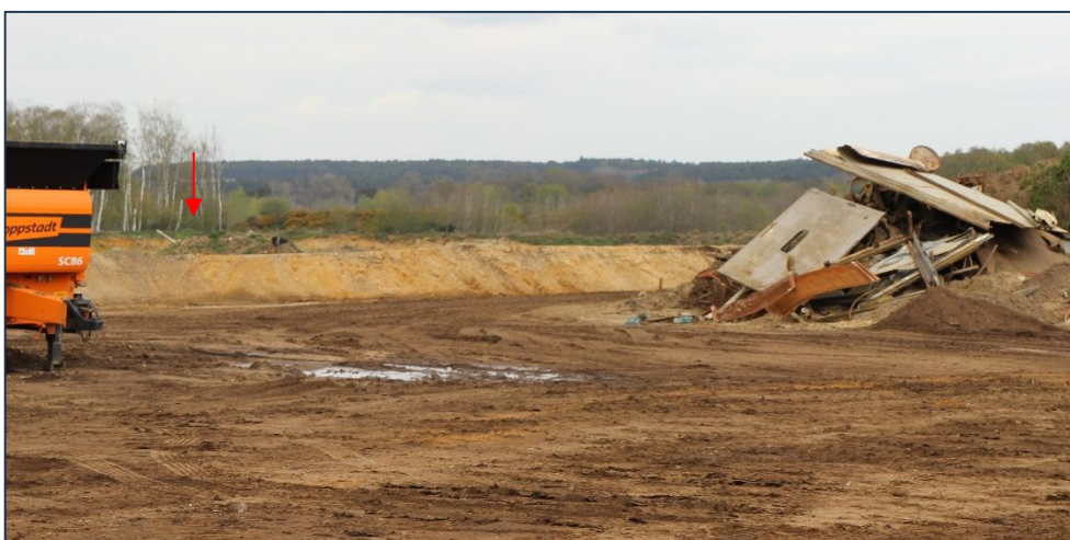
Figure 14 View towards Black Ditches (arrowed red) within tree belt from eastern side of PDA at photograph location 4
