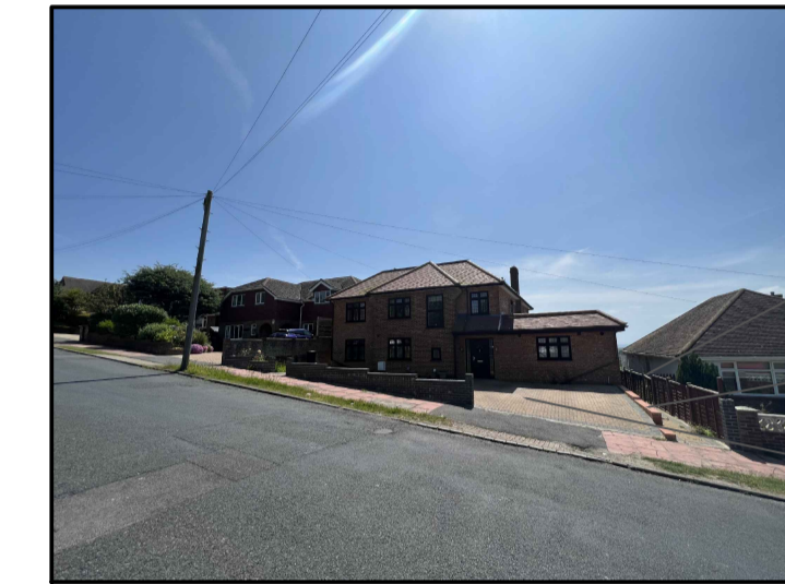
Access Gate Garden Wall Widened Driveway
