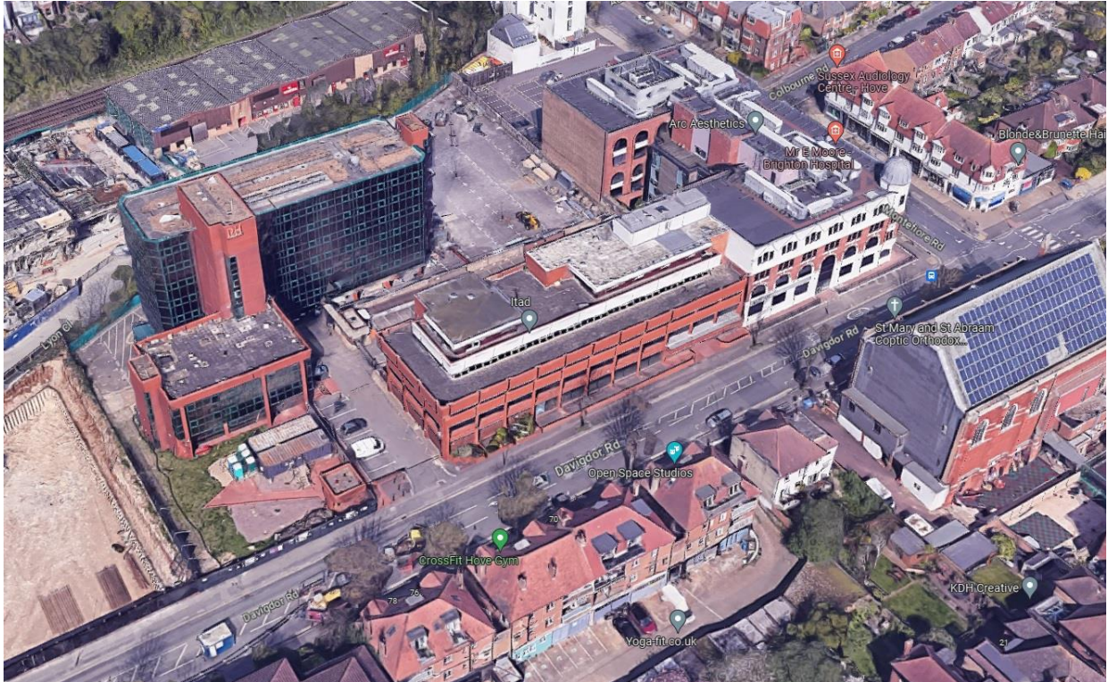
Figure 1 - Aerial photo of the Site and neighbouring buildings (© Google)
