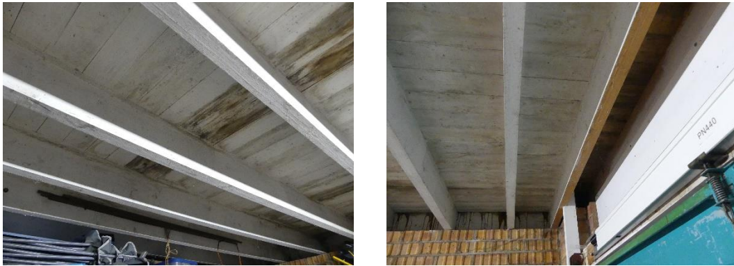
Figs. 18 & 19 Interior of garage
