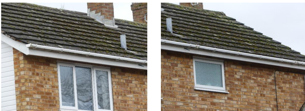
Figs. 4 & 5 Concrete tiled roof of house
