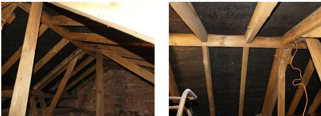
Figs. 14 & 15 Roof void of house
