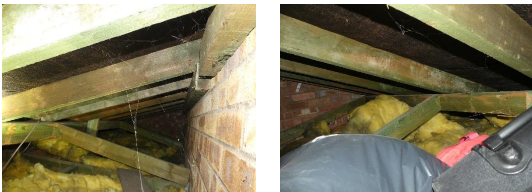
Figs. 16 & 17 Roof void of extension
