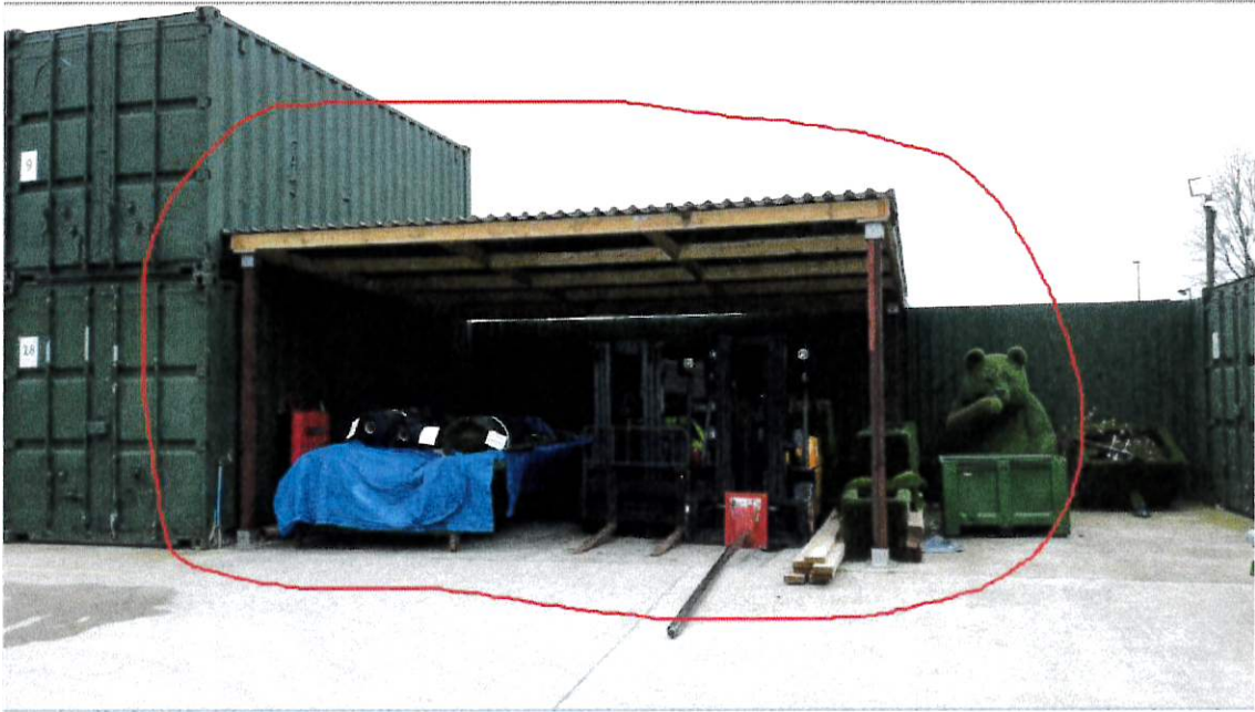
Flat Roofed Structure
