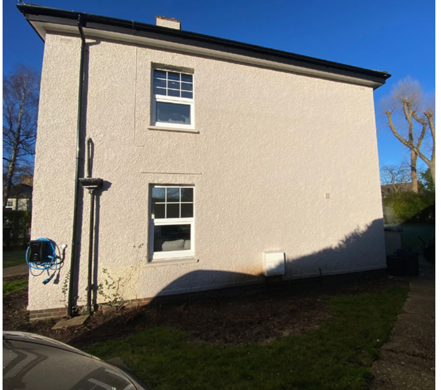
Existing flank facade
