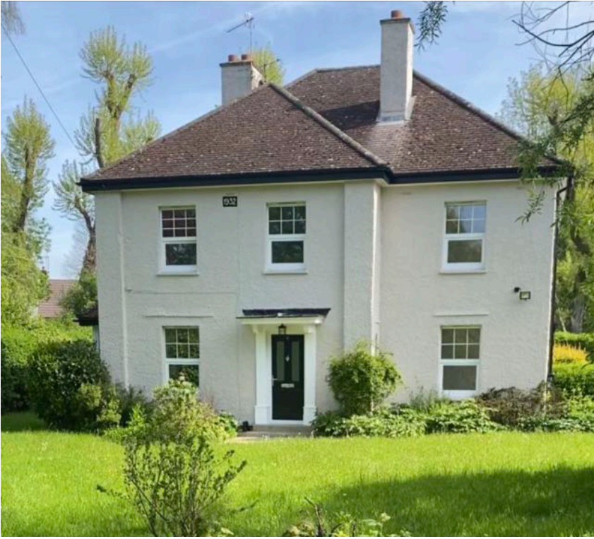
Existing front facade
