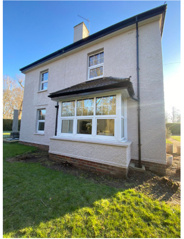
Existing flank facade
