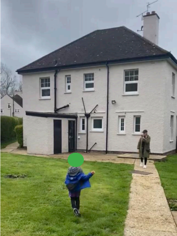
Existing rear facade
