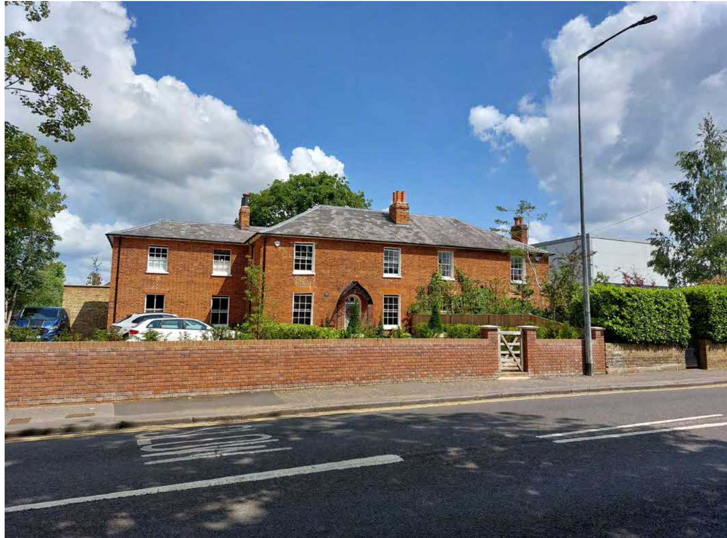
Figure 4.1 - Cromwell Cottage and Hill Cottage.
