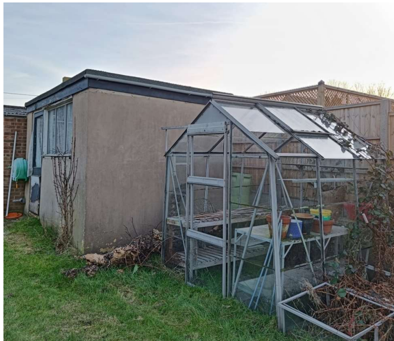
Fig. 6: Existing Outbuilding and greenhouse to the rear of the existing garage.
