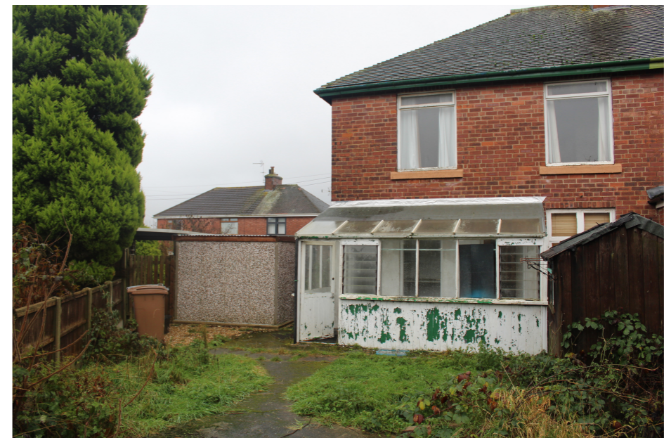
Image 3: View of rear elevation of existing building
