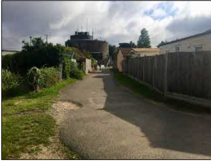
Fig 11: View from No 35 NE to Martello Tower, the entrance to the cul de sac.
