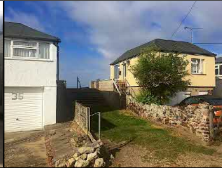
Fig 12: No 35 & No 36 showing the public access to the sea wall prom & Gate West 2.
