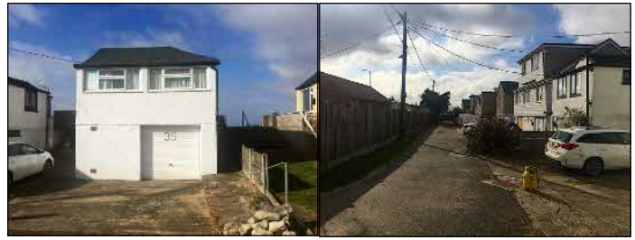
Fig 7 & 9: Views of No. 35 Tower Estate, Tower Estate Road. Front elevation showing two stories & car parking with seawall behind, and the view to the left (SE) along cul-de-sac showing Nos 36 to 42 on the right.
