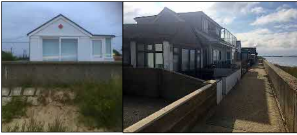
Fig 6 & 7: Views of No. 35 Tower Estate Rear elevation showing one habitable storey & front door, and the view to the right (South East) down the seawall promenade showing Nos 36 to 42.
