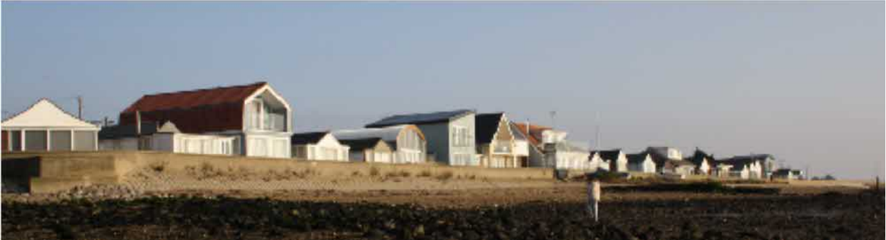
Fig 14: Photograph demonstrating the pattern of original short chalets and the newly build chalets all set behind the seawall.
