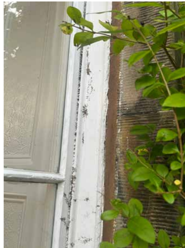
3. Flaking/rotting
