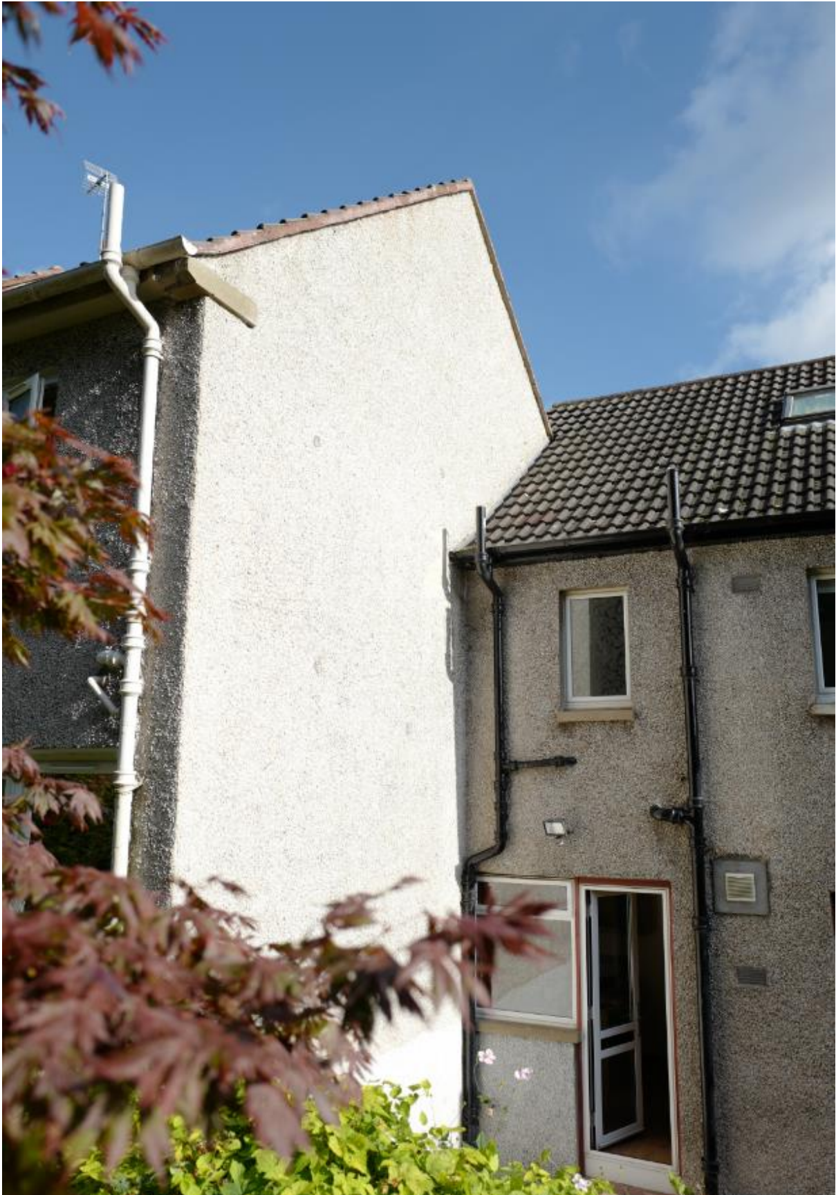
Fig 2: Step back shown on gable
