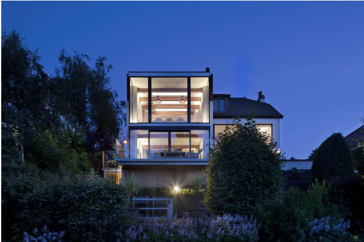
Fig 9: Remodelling and house extension in suburban Whitecraigs, David Blaikie Architects
