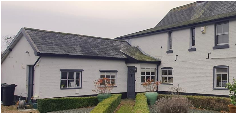
Lean to porch on rear extension
