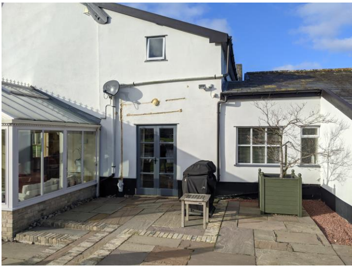
Photo 1 View of where the new extension is proposed (i)
