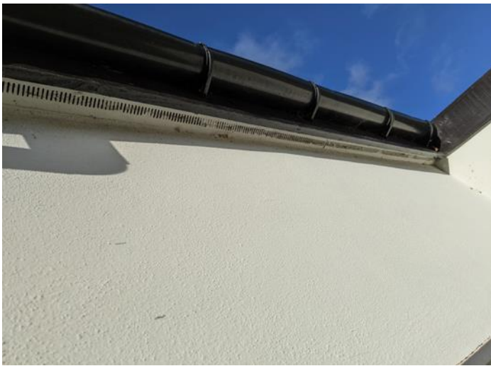
Photo 3 View of sealed soffits supporting no bat roosting potential
