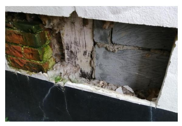
Sections of render have been removed to give some limited insight into the frame condition – the sole plate (if it still exists!) is under concrete and the infill panels appear predominantly modern. Any defective historic timbers will be repaired as appropriate using hidden splints and face-patches primarily but scarfs if required. Once the studs and posts have been repaired a new sole plate will be fitted in sections and the components pegged together.
