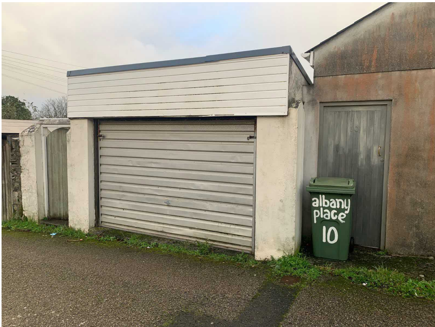
Figure 1: South-eastern elevation of garage
