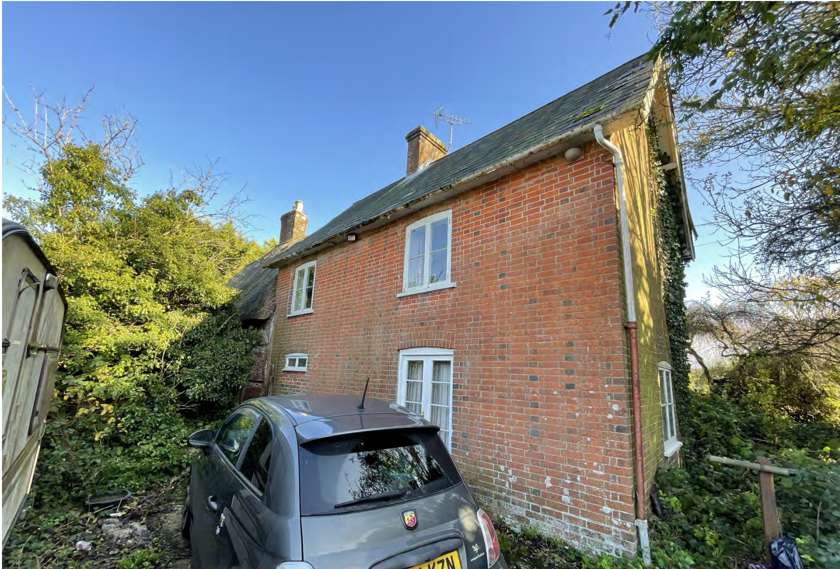
Plate 18: Old Farmhouse, two-storey brick and slate extension, west elevation.
