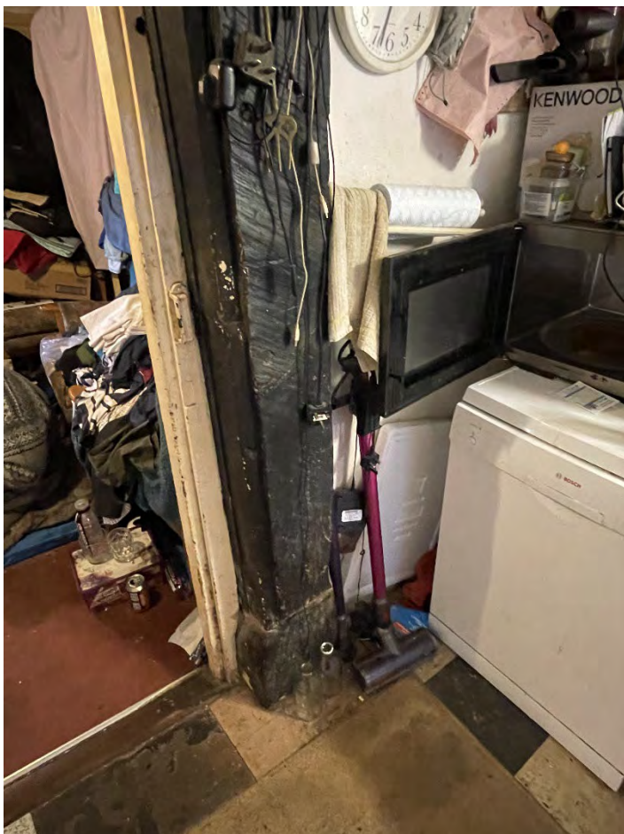
Plate 28: Old Farmhouse, detail of exposed timber frame on the ground floor.
