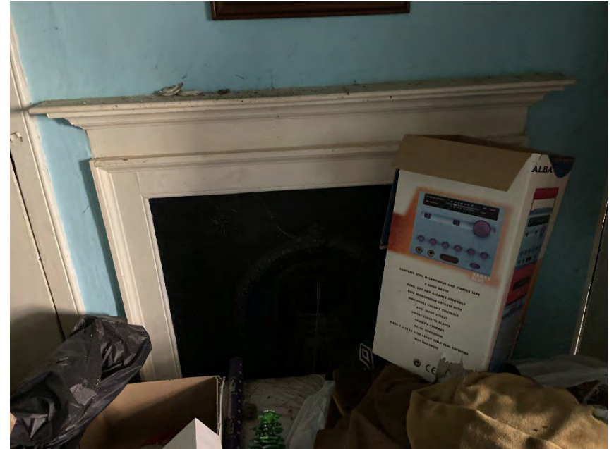
Plate 27: Old Farmhouse, moulded timber fireplace surround with cast iron inset on the first floor of the historic core.
