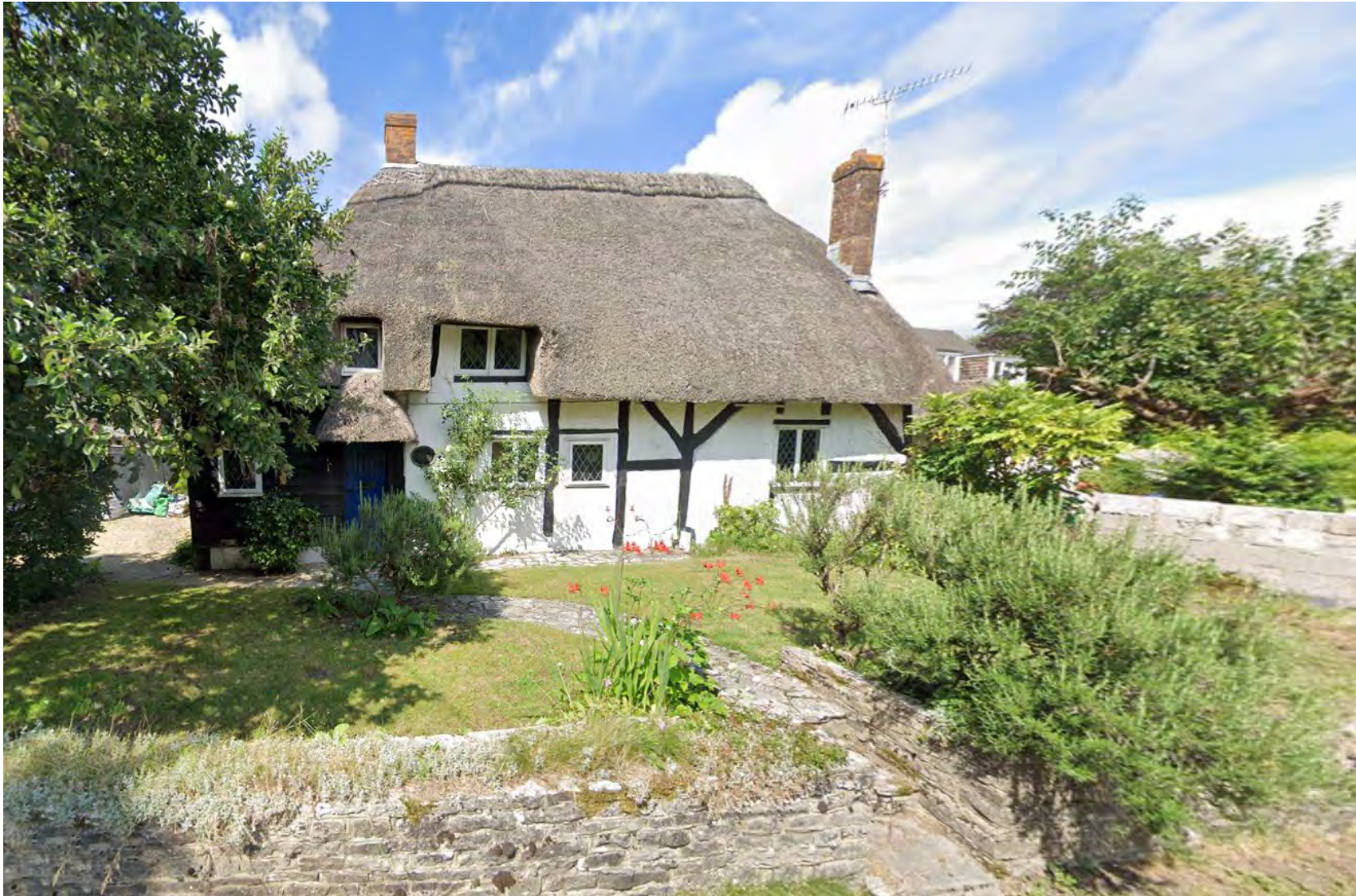
Plate 48: Rosemary Cottage, principal south elevation as seen from Fryern Court Road.
