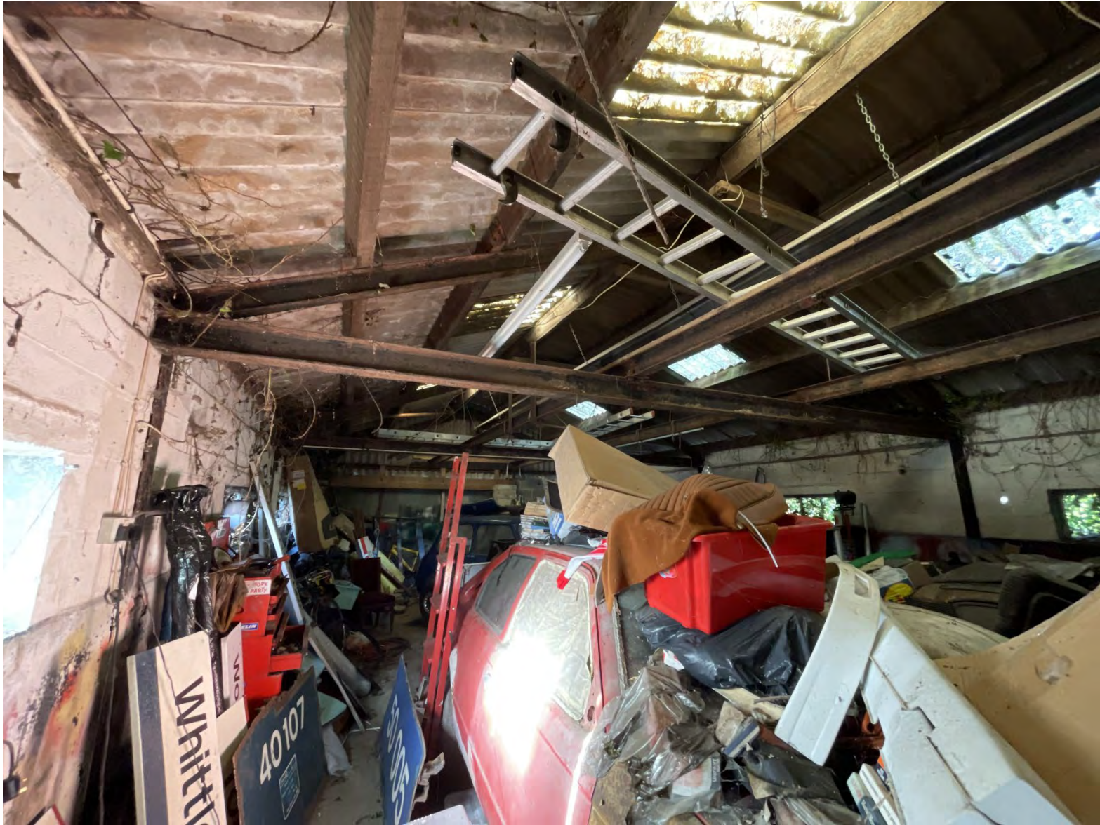
Plate 44: Building E, interior of barn/workshop.
