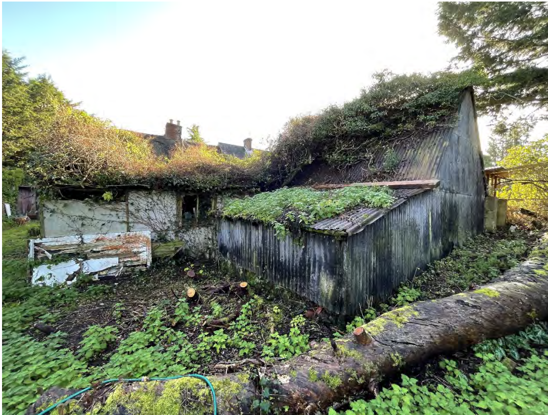
Plate 37: South-east-facing view of Buildings C and D.
