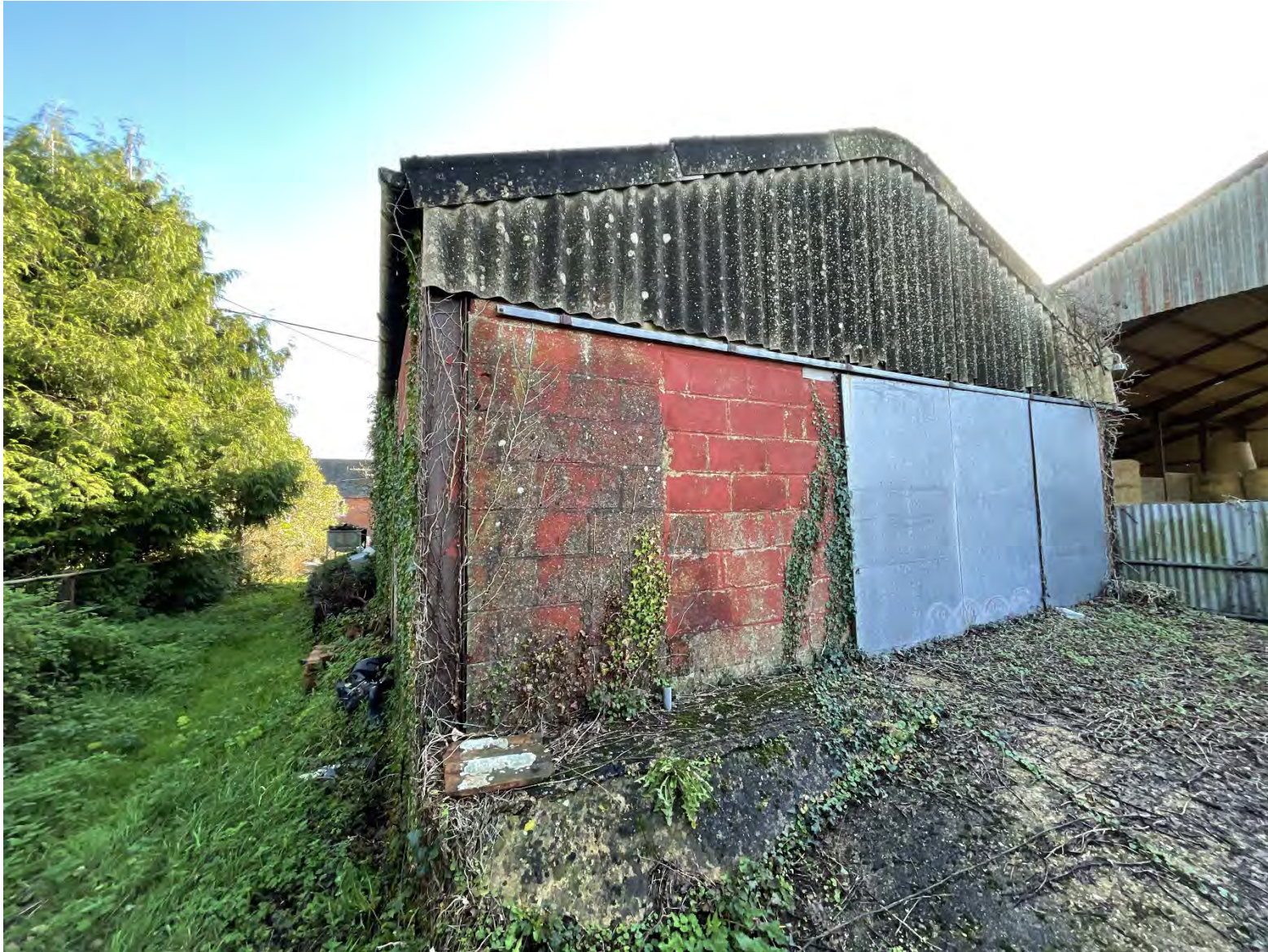
Plate 43: Building E, west elevation.
