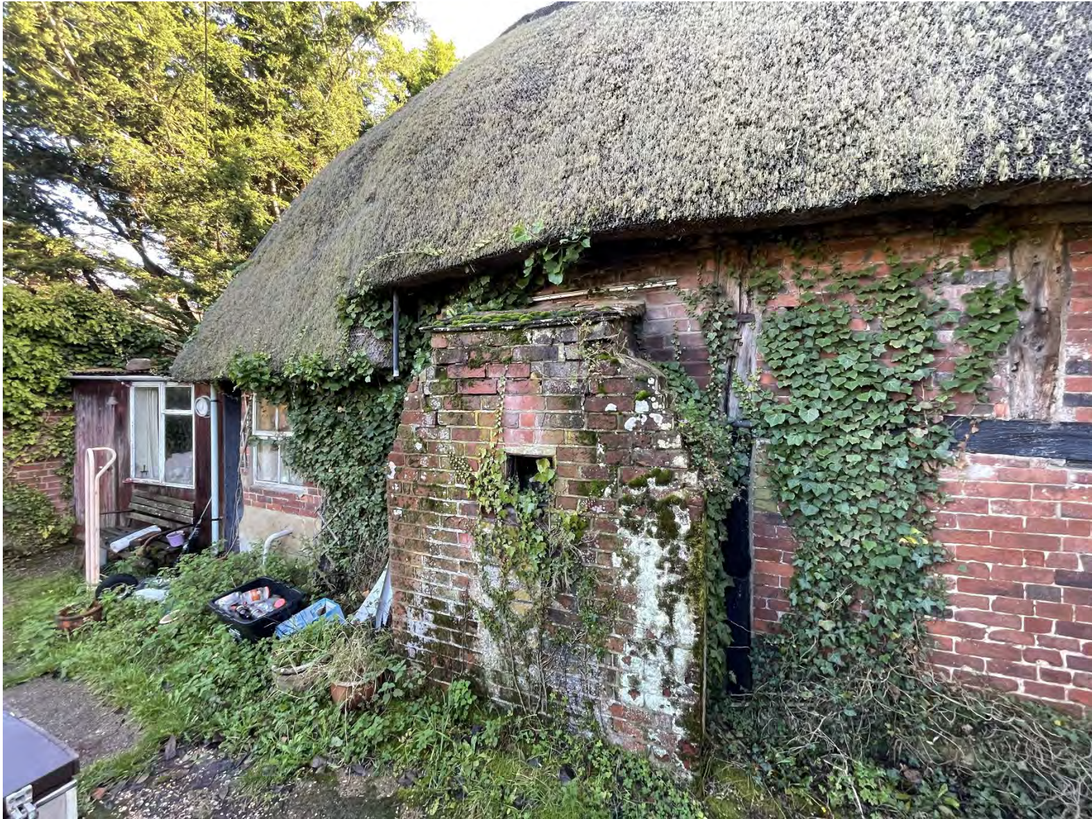
Plate 15: Old Farmhouse, west (rear) elevation, detail of north side.
