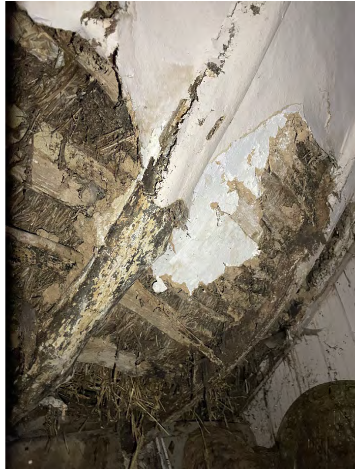
Plate 20: Old Farmhouse, detail of roof structure in the historic core.
