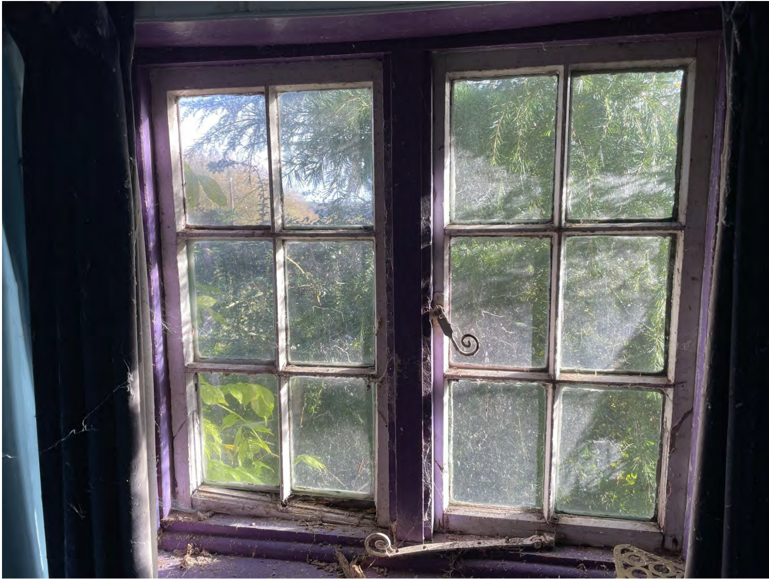
Plate 23: Old Farmhouse, example of first-floor window.
