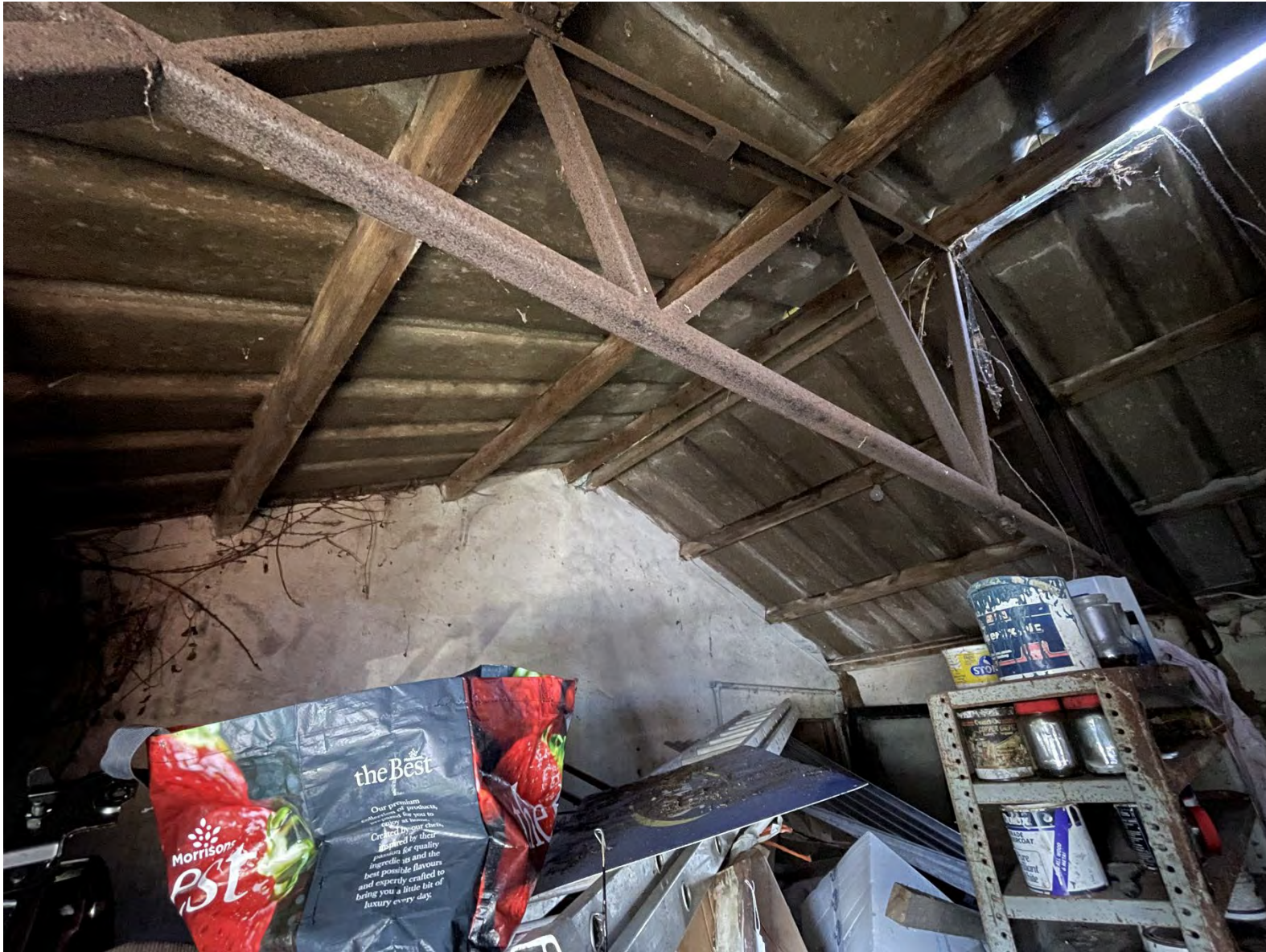
Plate 42: Building E, interior of east range.
