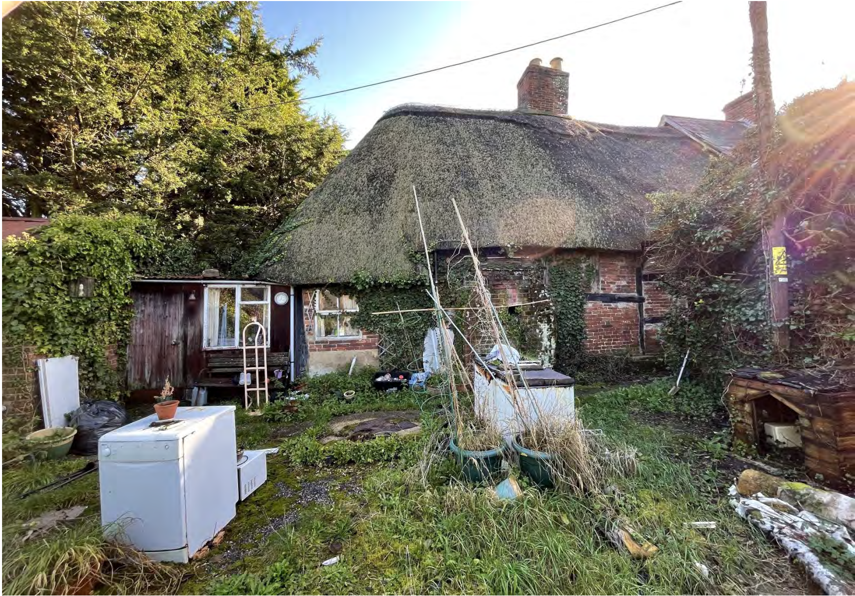
Plate 13: Old Farmhouse, west (rear) elevation.
