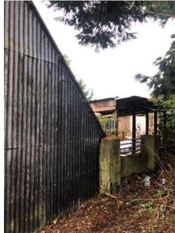
Fig 5 & 6: Views of existing outbuilding (Building 2)
