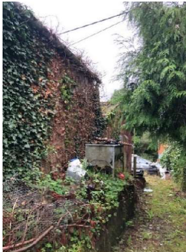
Fig 7 & 8: Views of the existing outbuilding (Building 3)
