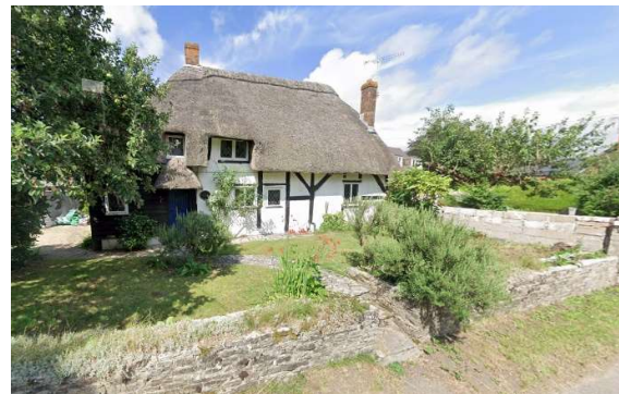
Fig:14 Rosemary Cottage, Grade II Listed Entry No. 1301254
