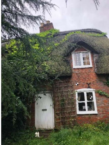
Fig 11: Old Farmhouse, Grade II Listed Entry No. 1181378
