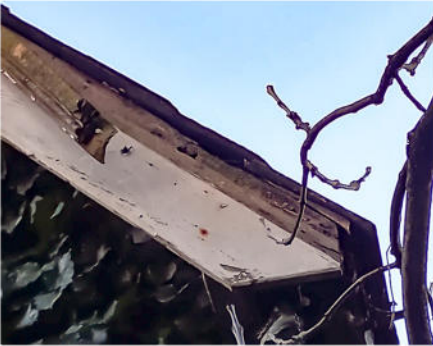
Photo 5: Displaying areas of lifted tiles on the western aspect of building B1.
