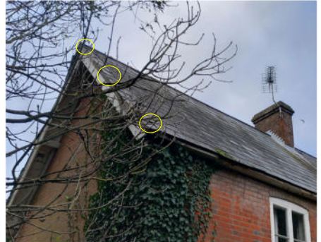
Photo 6: Displaying lifted roof tiles on the eastern aspect of building B1.
