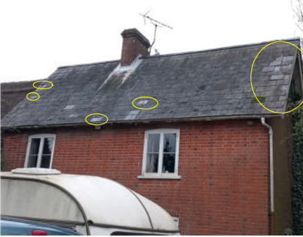
Photo 5: Displaying areas of lifted tiles on the western aspect of building B1.
