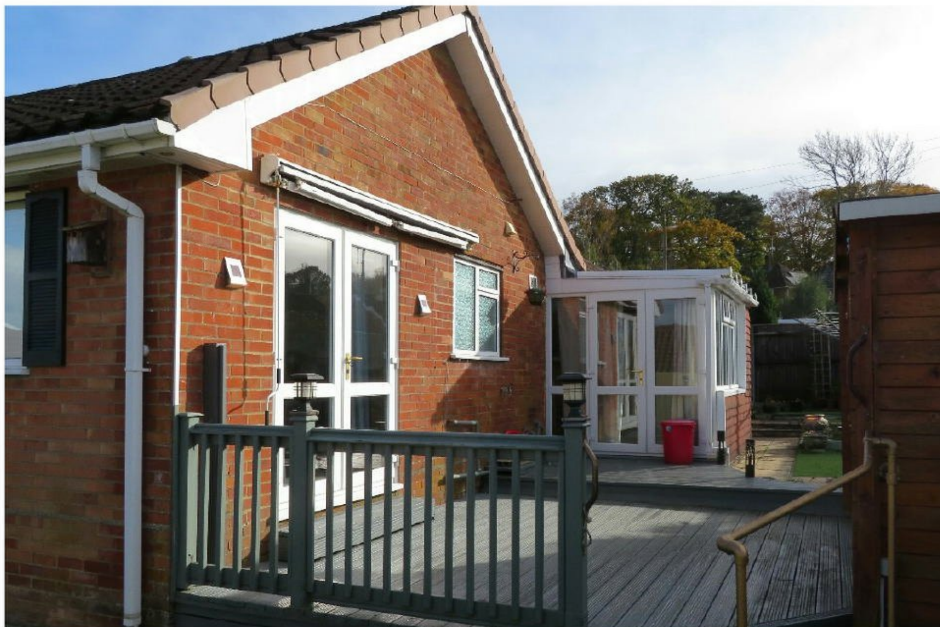
Photo viewing Part Rear / Side of Property from Back Garden (Camera Facing South East)
