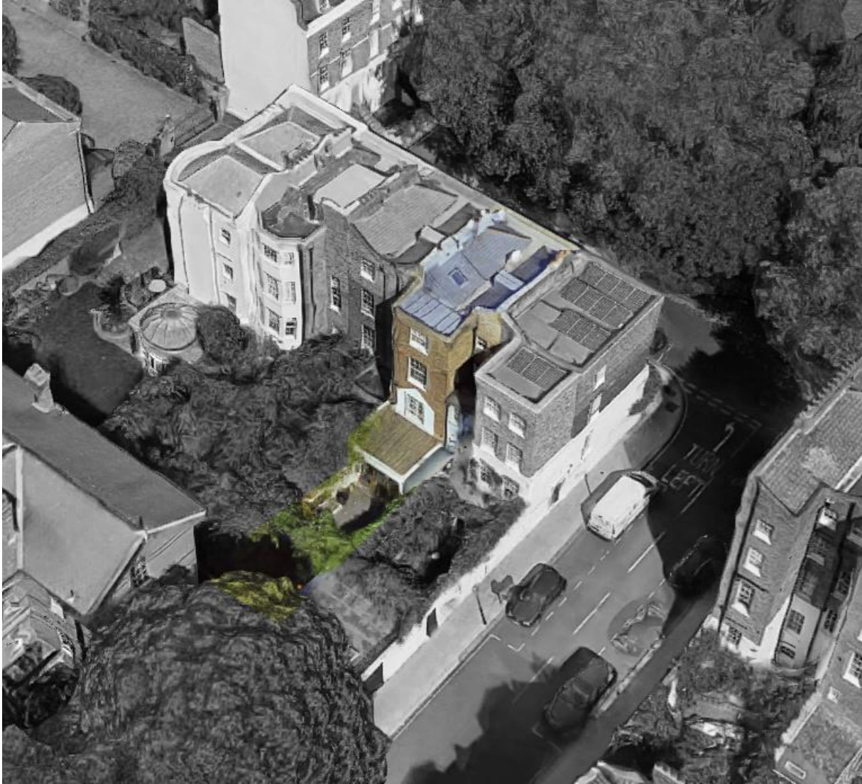
AERIAL VIEW Source: Google Maps
