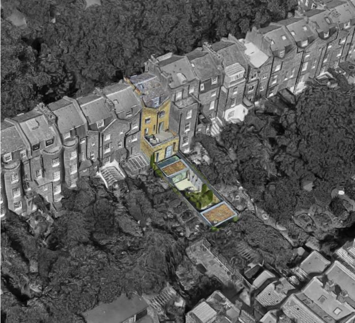
AERIAL VIEW Source: Google Maps
