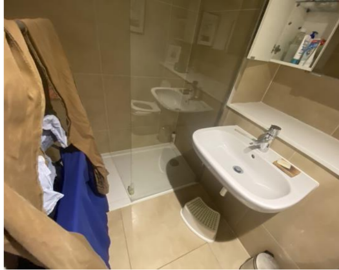
LOWER GROUND FLOOR SHOWER ROOM
