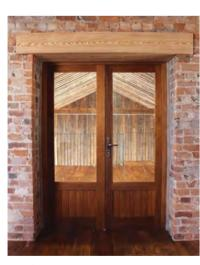
Note: New Master Suit Walk in Wardrobe knock through stone wall and add oak beam lintels to create 2100mm x 900mm opening. solid wall comes through from the ground floor to roof level into the roof area.
