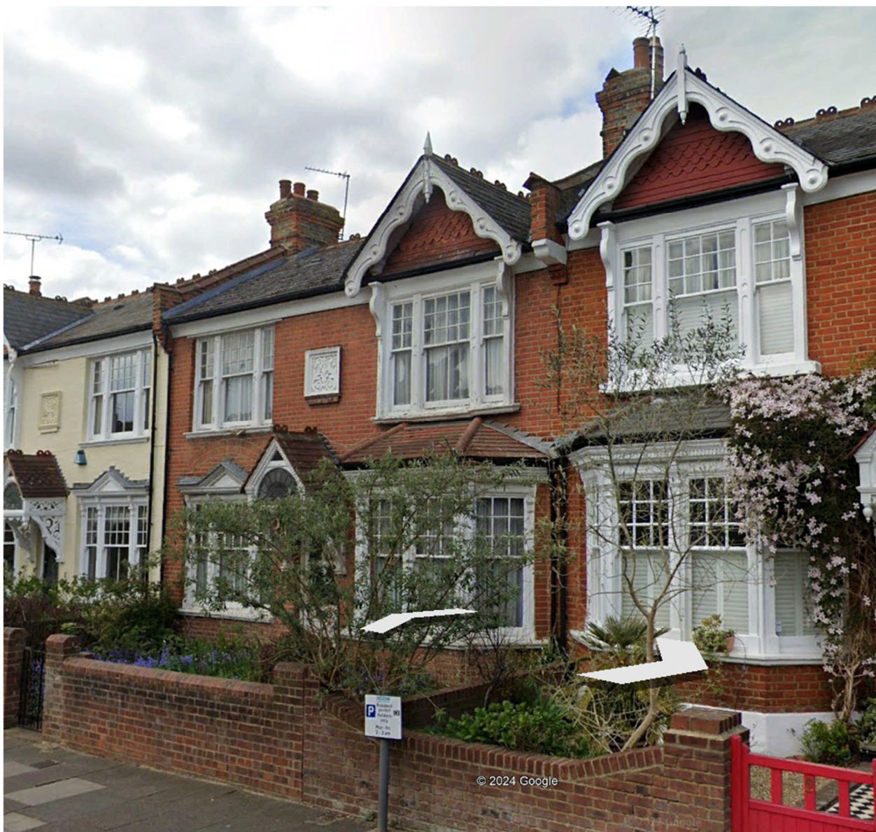
View from the road of terrace of three house with No.4 Duke Avenue in the center.
