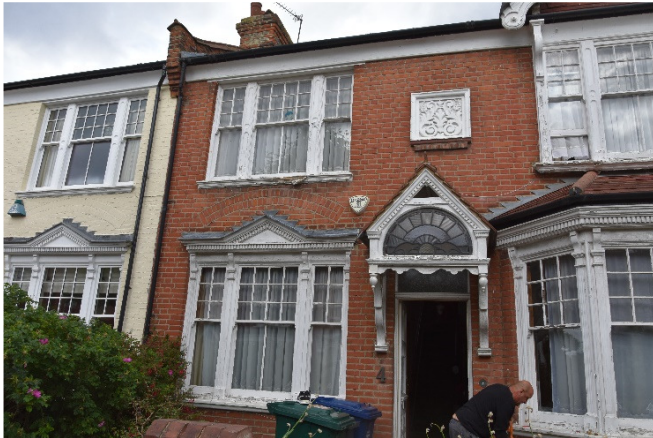
Existing central entrance with reception rooms either side.
