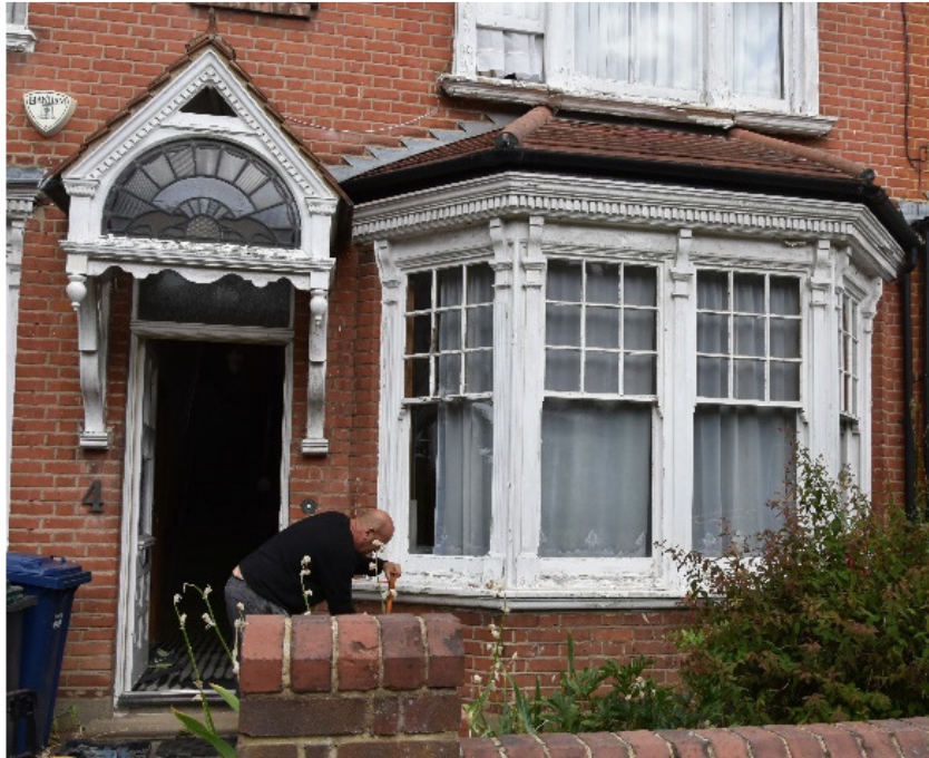
The ornate bay window and entrance canopy have deteriorated due to lack of maintenance
