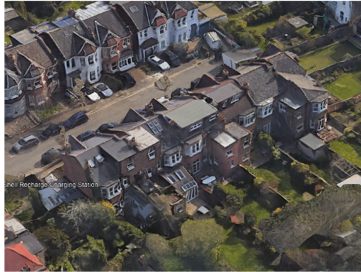
Far end of Dukes Avenue with extensions to North side in the foreground.
