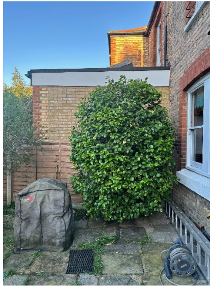
Extension at No.2 from No.4 garden.
