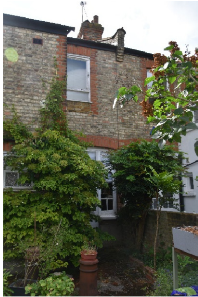
Recessed area of rear elevation.
