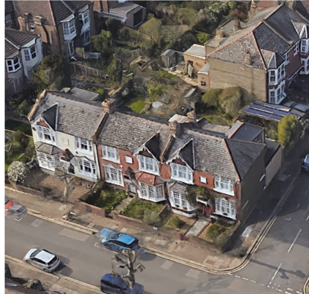
Aerial view of front of No.2, 4 & 6 Dukes Avenue.
