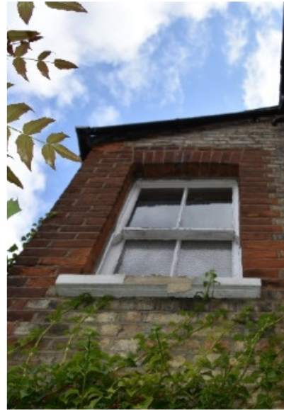
Side window overlooking extension area.
