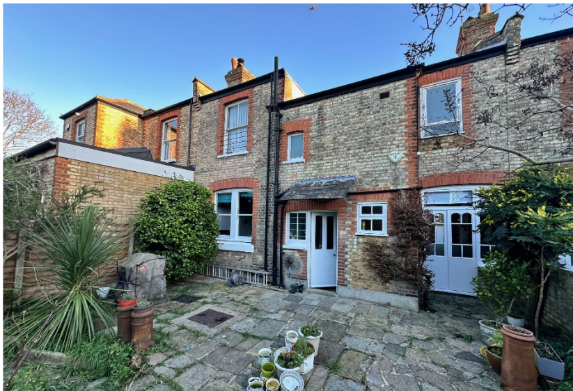
Rear elevation with extension at No2 on the left-hand side.
