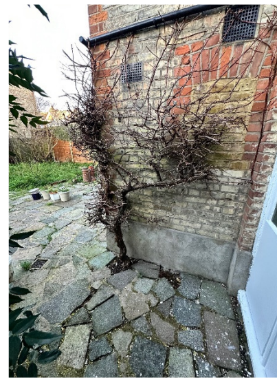
Flank wall to ground floor wc.
