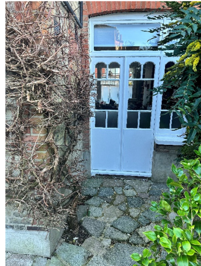
Flank wall to ground floor wc.
